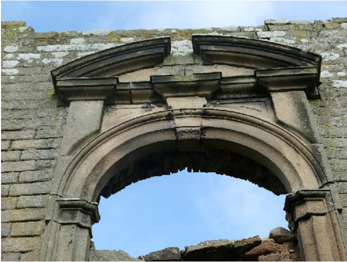
Figure 24. Pavilion or tea-house. Detail of a window opening showing oak leaf decoration on the keystone of the arch.
