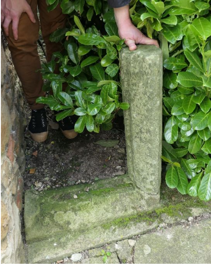
Figure 34. Sill and mullion of window from the Jacobean house re-used in a rockery.
