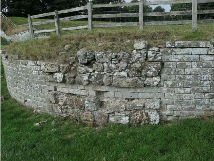
Figure 19. Bands of rusticated masonry in the half-moon bastion.
