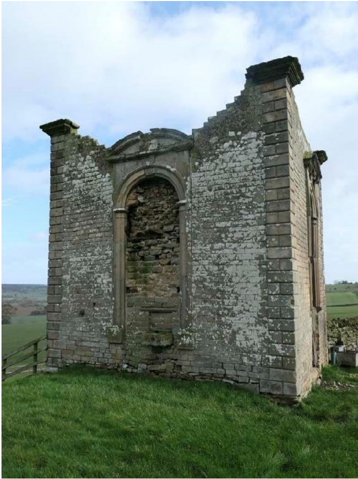
Figure 23. The blocked doorway of the 'Bell Park' pavilion or tea-house.
