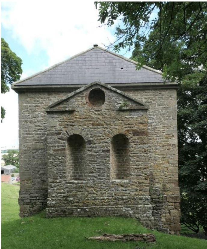
Figure 28. 'Summer house', rear view.
