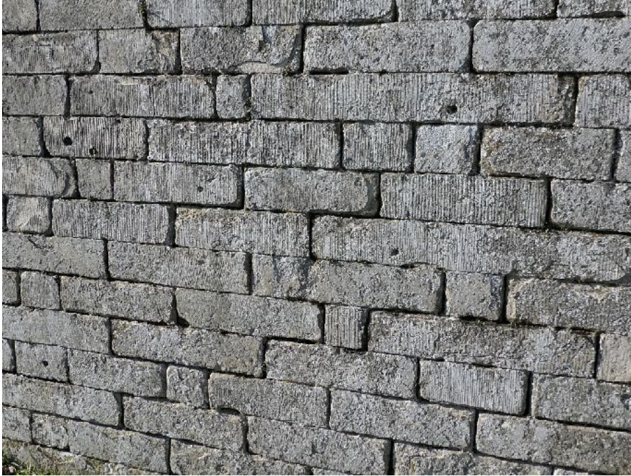
Figure 18. Ridged tooling on the ashlar masonry of the bastioned wall.
