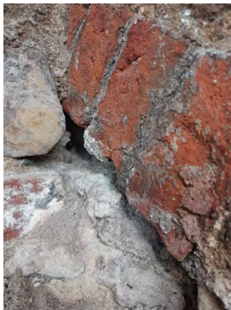
Detail of the fragment of arch at the junction between the north and west walls
