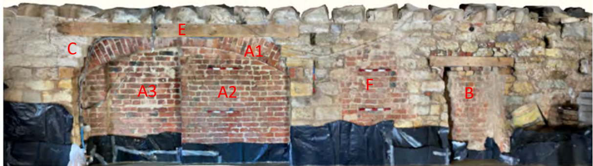
The west wall showing the positions of features referred to below
