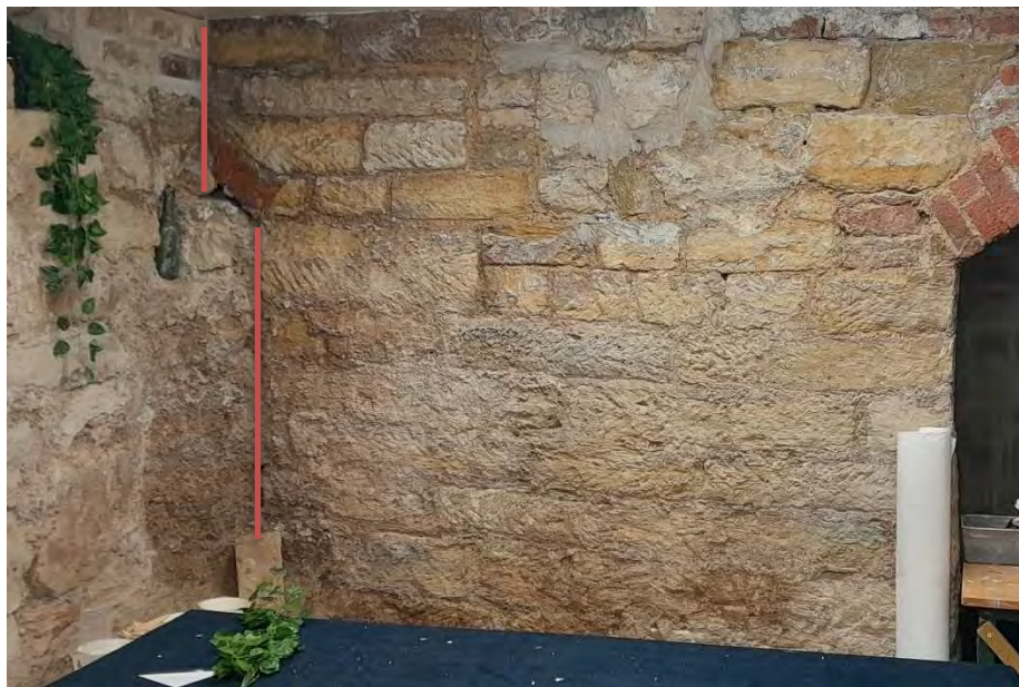
The west end of the north wall at its junction with the side wall showing the small section of visible brick arch abutted by the later side wall. Straight joints are indicated by the red lines
