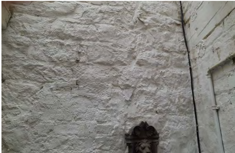
Fragment of stone wall in the yard of 98 Castle Road
