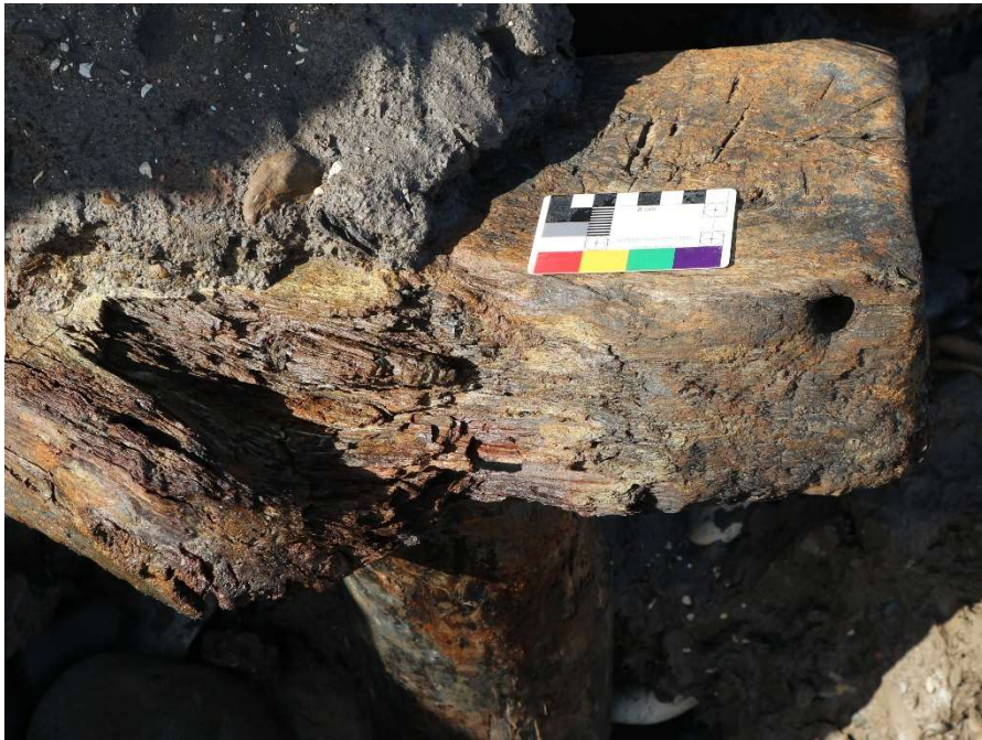
Figure 5 Close detail of the horizontal beam showing the peg hole
