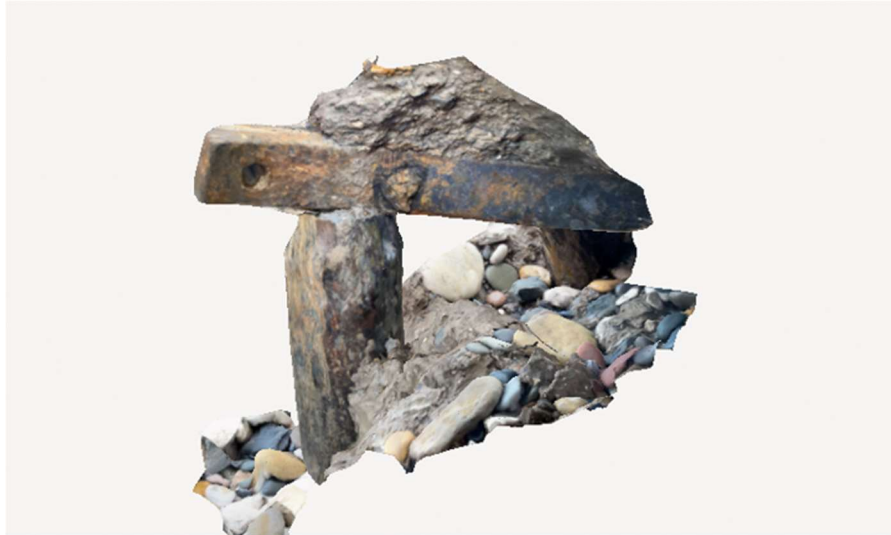
Figure 6 Detail of the rear of the beam showing the peg hole and possible iron bolt
