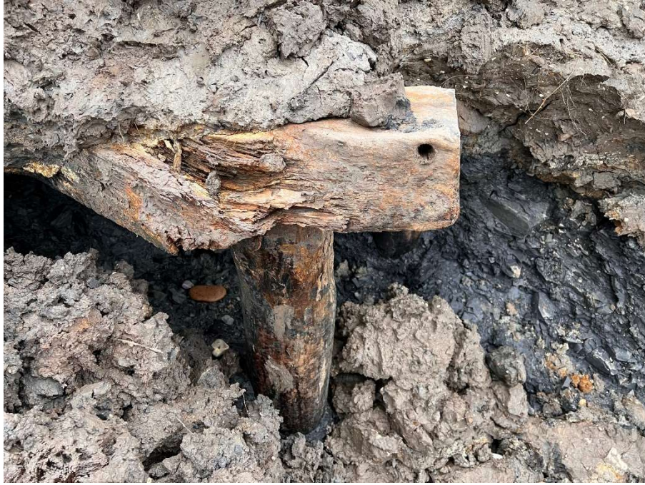
Figure 4 Post 3 showing details of the horizontal beam
