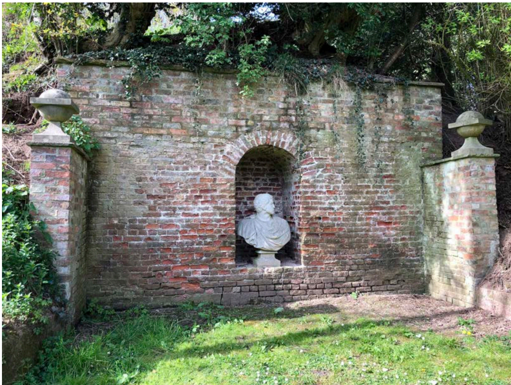
Figure 11. The brick niche.
